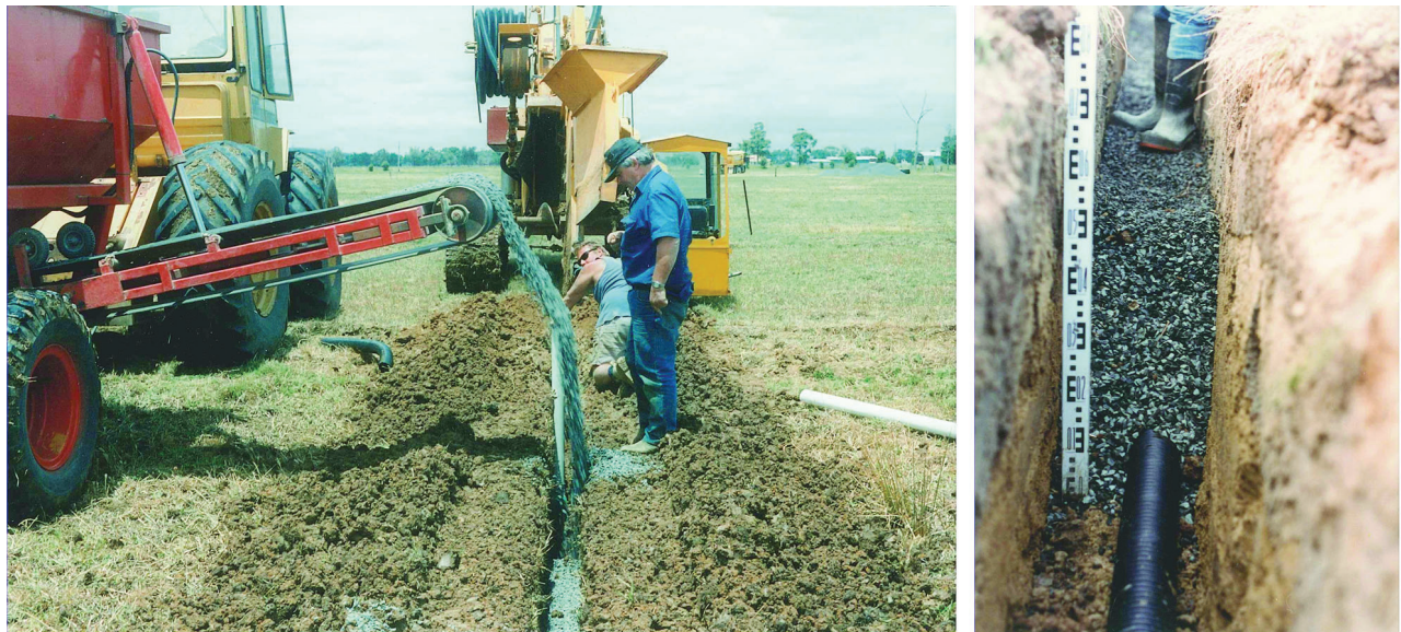
Figure 13 Installing a main French drain. (Skilled Trades BC, 2021; Western Australian Agriculture Authority) WAAA Copyright ( https://www.agric.wa.gov.au/copyright )
