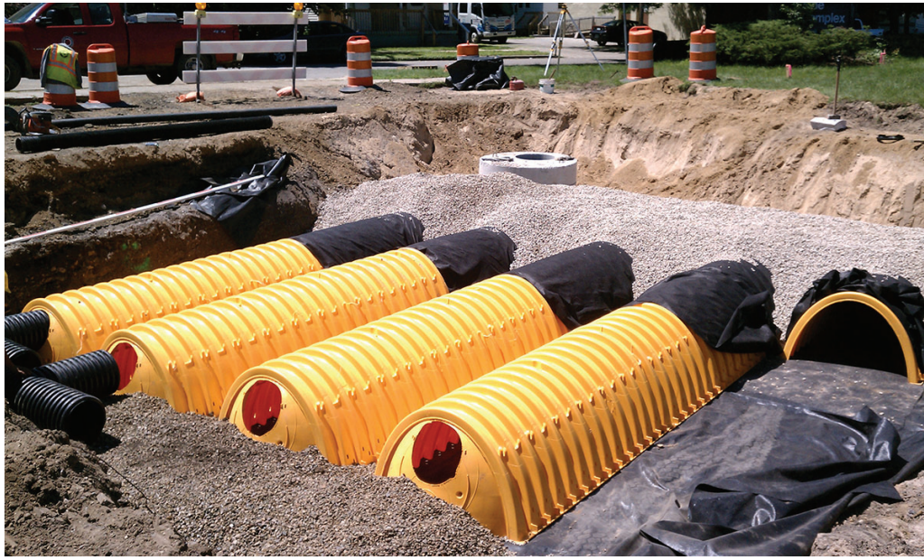
Figure 3 Arched infiltration chambers. (Arbitrarily0/Wikimedia Commons) CC BY-SA 3.0 ( https://creativecommons.org/licenses/by-sa/3.0/deed.en )
