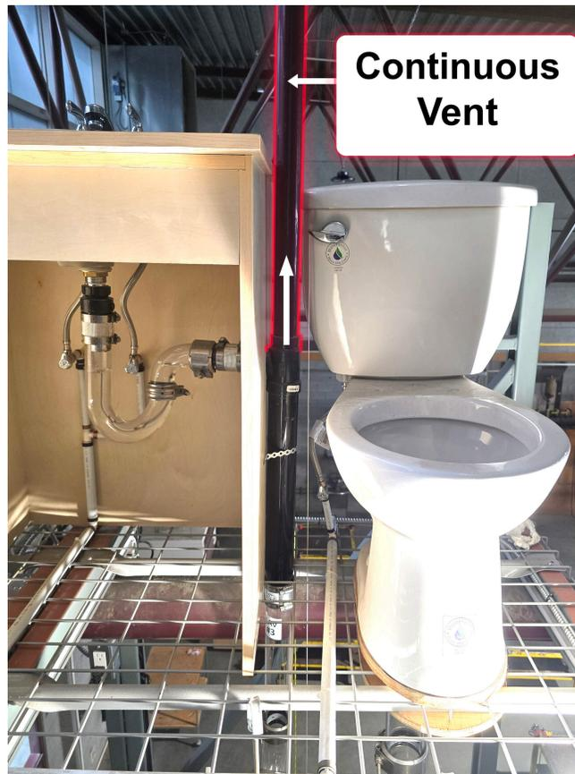
**Figure 11** Continuous vent. (TRU Open Press). CC-BY-NC-SA (<https://creativecommons.org/licenses/by-nc-sa/4.0/deed.en>)
