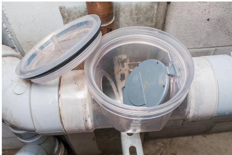
**Figure 4** Backwater valve. (Skilled Trades BC, 2021) Used with permission.
