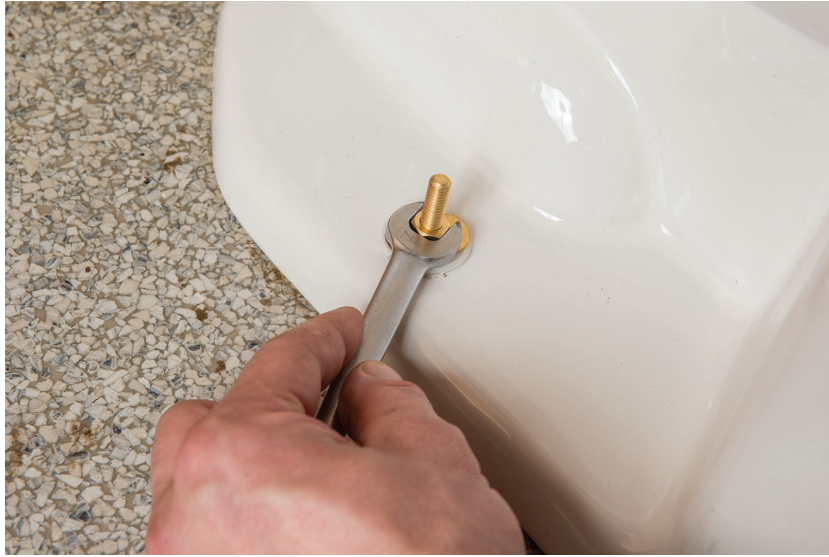
Figure 29 Tighten nuts. (Skilled Trades BC, 2021) Used with permission.
