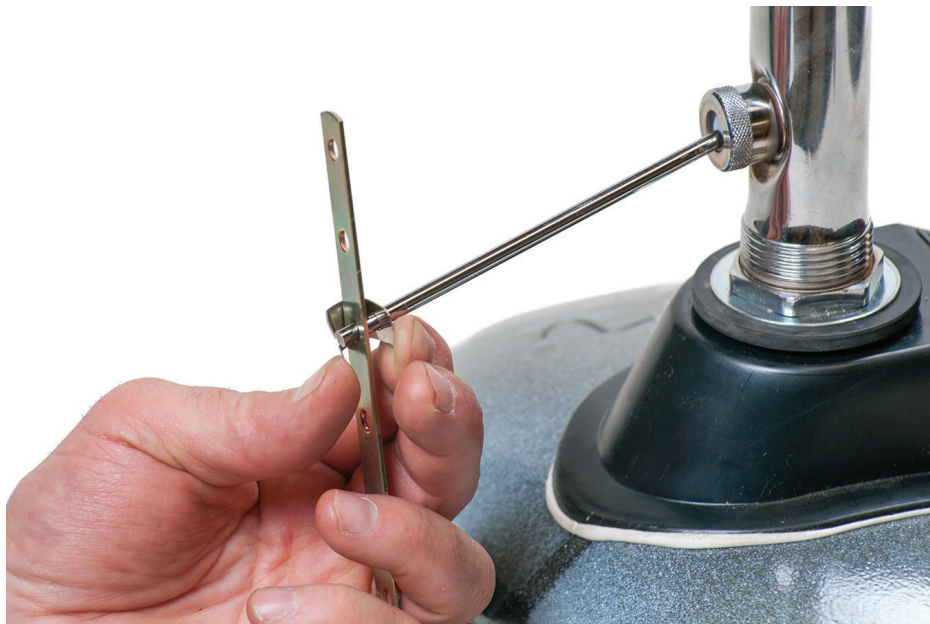
Figure 19 Squeeze clip gently. (Skilled Trades BC, 2021) Used with permission.
