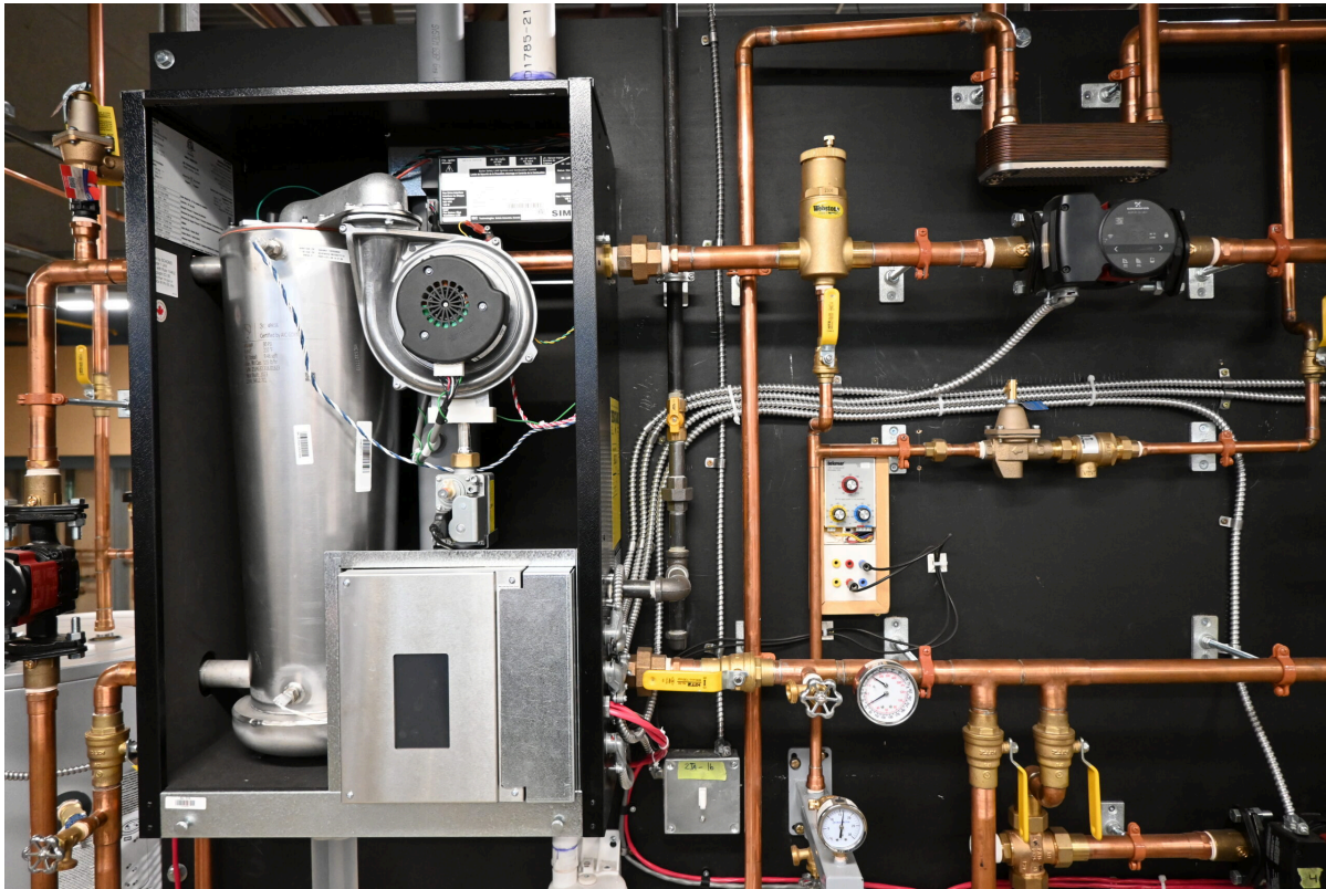
Figure 9 Wall-hung boiler service valves. (TRU Open Press) CC BY NC SA ( https://creativecommons.org/licenses/by-nc-sa/4.0/deed.en )
