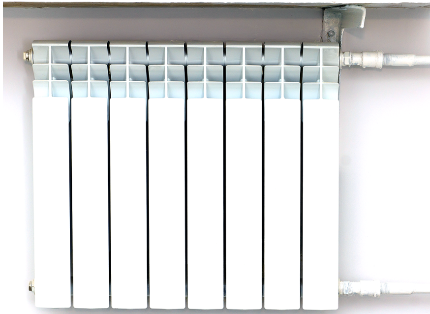
Figure 13 Wall-mounted panel radiator. (Skilled Trades BC, 2021) Used with permission.
