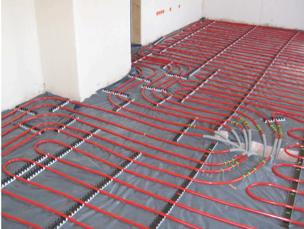
Figure 14 Radiant floor panel. (H. Raab (User:Vesta)/Wikimedia Commons) CC BY-SA 3.0 ( https://creativecommons.org/licenses/by-sa/3.0/deed.en )
