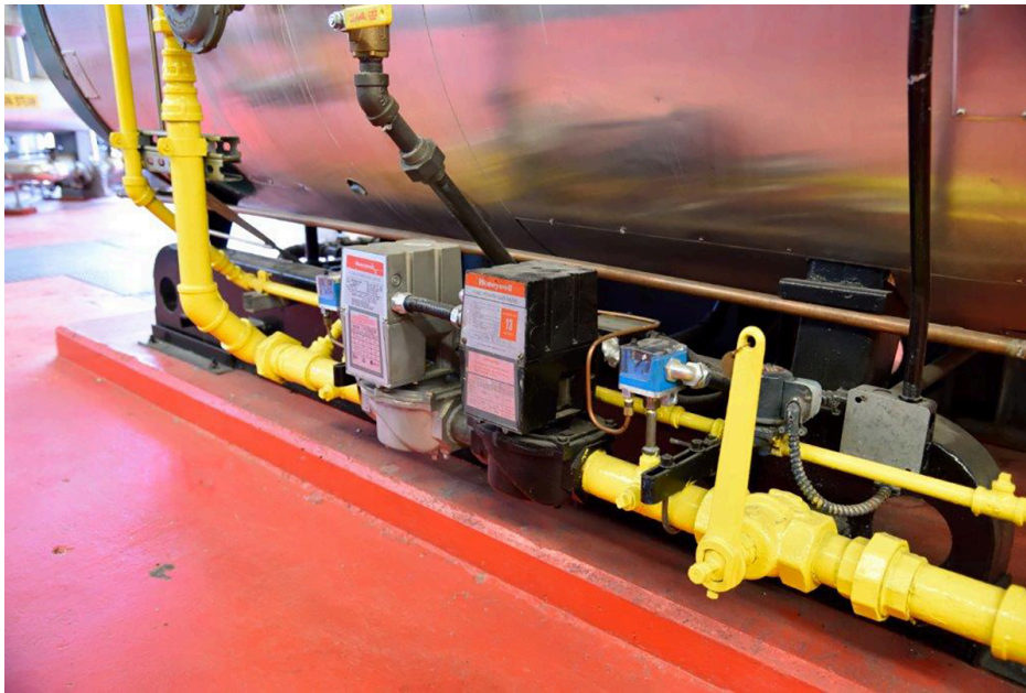
Figure 1 Industrial boiler mounted on housekeeping pad. (Skilled Trades BC, 2021) Used with permission.
