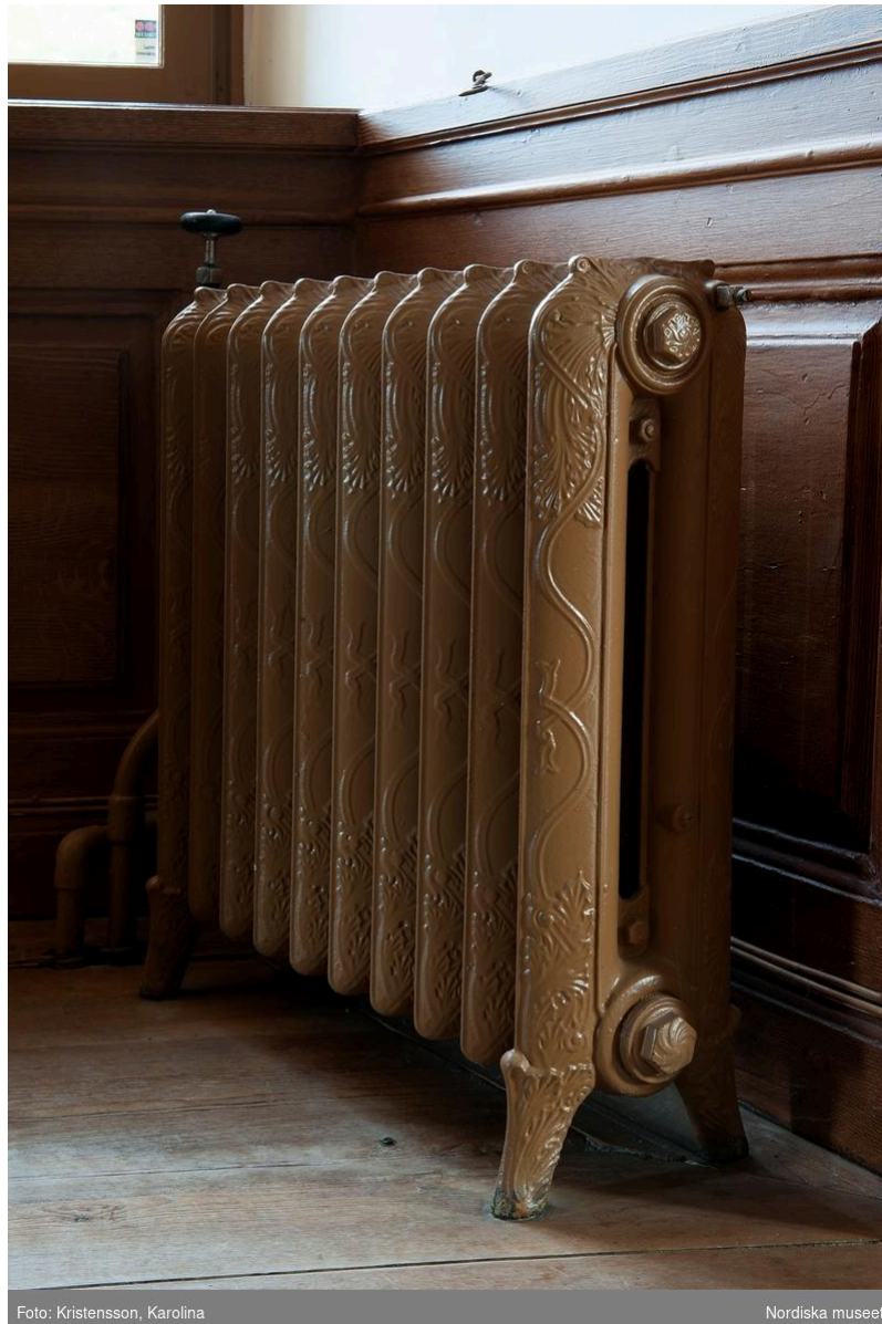
Figure 1 An installed freestanding cast-iron radiator. (Karolina Kristensson/DigitaltMuseum) CC BY-NC-ND 4.0 ( https://creativecommons.org/licenses/by-nc-nd/4.0/deed.en )
