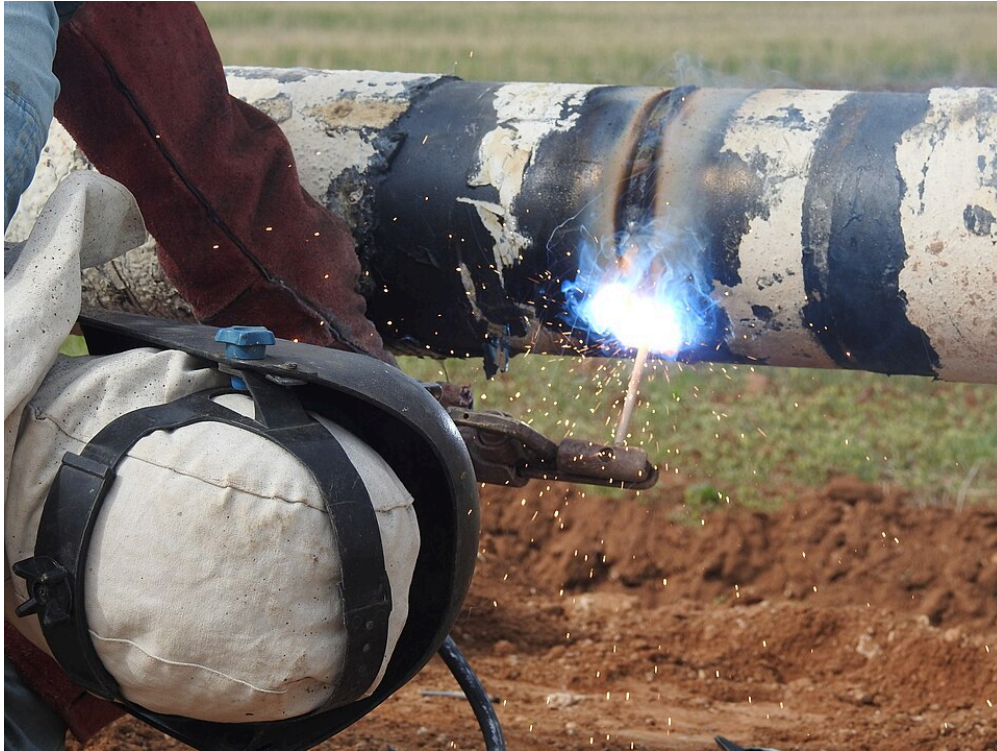
Figure 2 Gas pipeline welding (Hamid Soufi/Wikimedia Commons) CC BY-SA 3.0 ( https://creativecommons.org/licenses/by-sa/3.0 )
