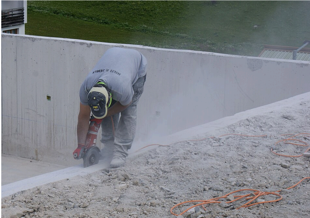
Figure 13 Angle grinder on concrete (Asumnupal/Wikimedia Commons) CC BY-SA 4.0 ( https://creativecommons.org/licenses/by-sa/4.0/ )
