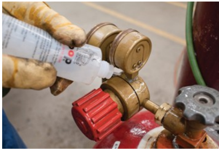
Figure 3 Apply a soapy solution to locate leaks (BC Industry Training Authority, 2019). CC BY-NC-SA 4.0 ( https://creativecommons.org/licenses/by-nc-sa/4.0/ )
