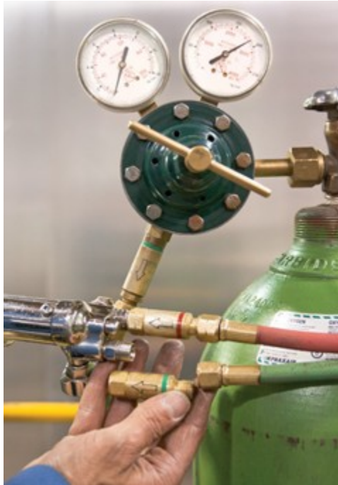
Figure 2 Installation of RFCVs (BC Industry Training Authority, 2019). CC BY-NC-SA 4.0 ( https://creativecommons.org/licenses/by-nc-sa/4.0/ )
