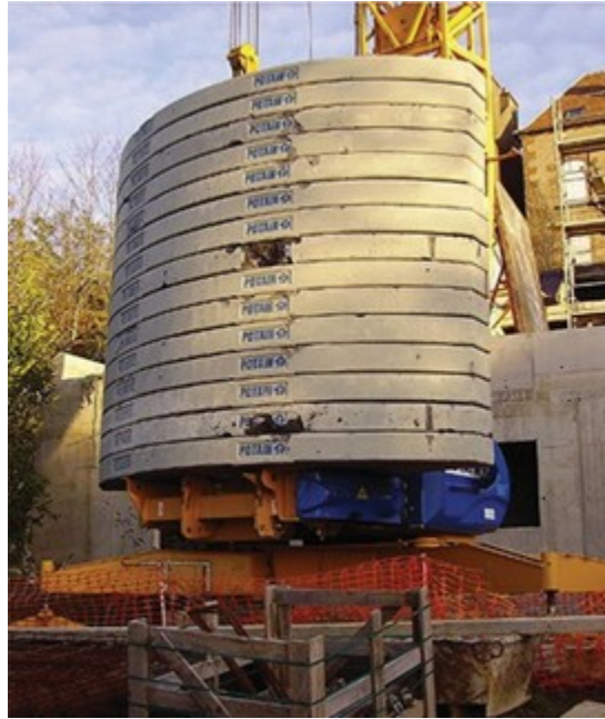
Figure 2 Counterweights (Cjp24/Wikimedia Commons) CC BY-SA 3.0 ( https://creativecommons.org/licenses/by-sa/3.0/deed.en )
