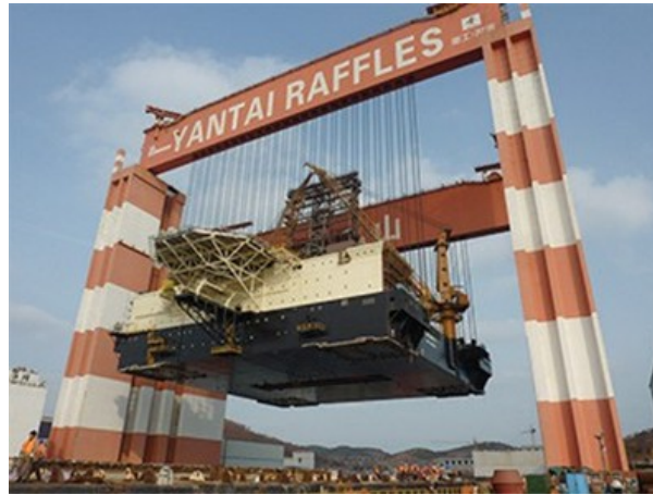
Figure 4 Gantry crane (Haakman/Wikimedia Commons) CC BY 3.0 ( https://creativecommons.org/licenses/by/3.0/deed.en ).
