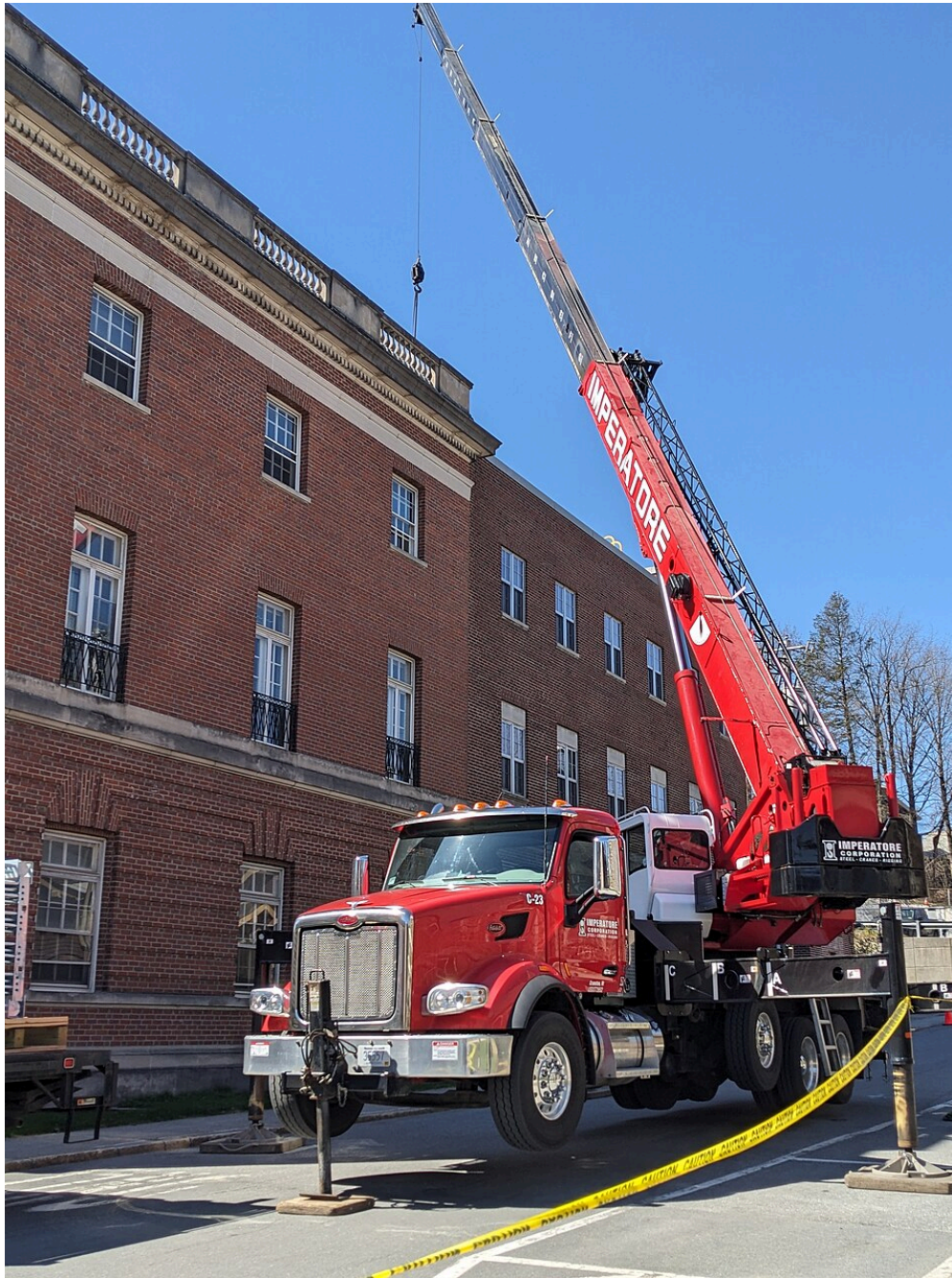
Figure 50 Boom truck in action (Artaxerxes/Wikimedia Commons) CC BY 4.0 ( https://creativecommons.org/licenses/by/4.0/deed.en )
