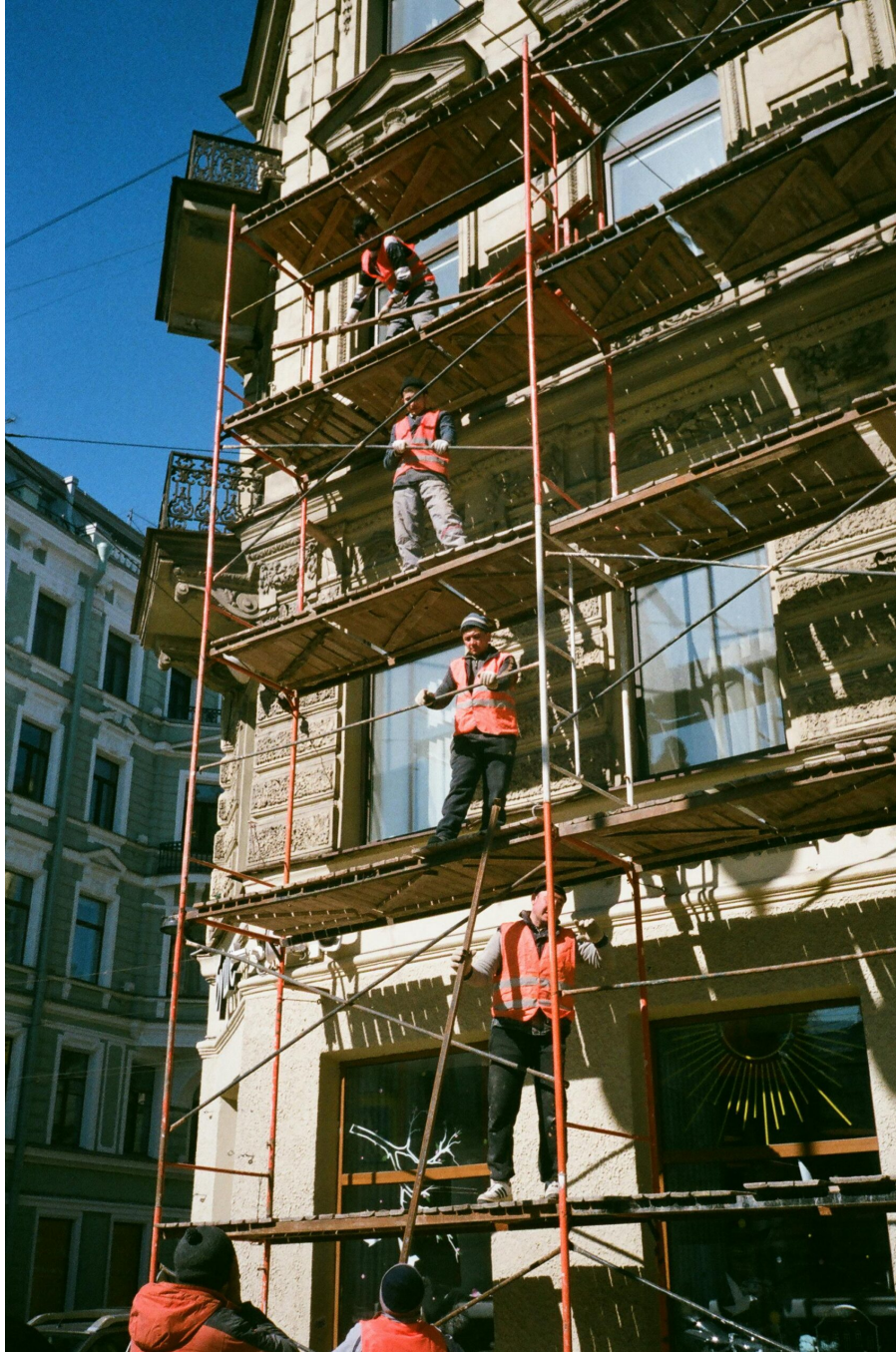
Men on Brown Scaffolding ( https://www.pexels.com/photo/men-on-brown-scaffolding-2209529/ ) (Darya Sannikova/pexels) Pexels License ( https://www.pexels.com/license/ )
