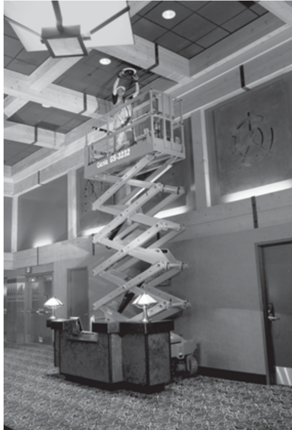
Figure 20 Scissor lift (elevated work platform) (BC Industry Training Authority, 2019). CC BY-NC-SA 4.0 ( https://creativecommons.org/licenses/by-nc-sa/4.0/ )
