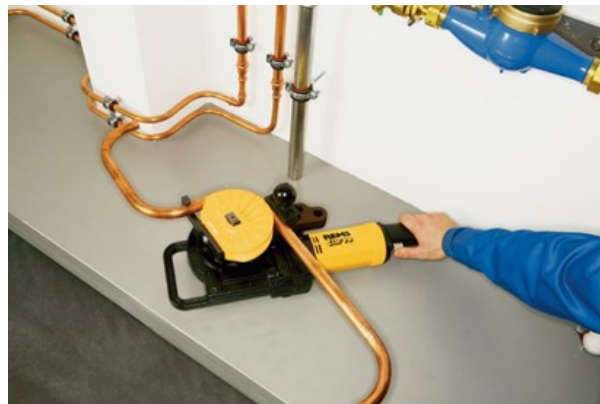
Figure 53 Portable power tubing bender in use (BC Industry Training Authority, 2019). CC BY-NC-SA 4.0 ( https://creativecommons.org/licenses/by-nc-sa/4.0/ )
