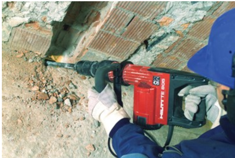
Figure 16 Demolition hammer or jack hammer (BC Industry Training Authority, 2019). CC BY-NC-SA 4.0 ( https://creativecommons.org/licenses/by-nc-sa/4.0/ )
