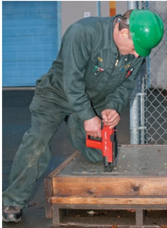
Figure 22 Using a powder-actuated tool (BC Industry Training Authority, 2019). CC BY-NC-SA 4.0 ( https://creativecommons.org/licenses/by-nc-sa/4.0/ )
