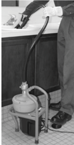
Figure 56 Sink machine cleaning a fixture drain (BC Industry Training Authority, 2019). CC BY-NC-SA 4.0 ( https://creativecommons.org/licenses/by-nc-sa/4.0/ )
