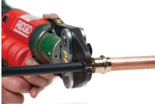
Figure 109 Copper x PEX press-fit adapter (BC Industry Training Authority, 2019). CC BY-NC-SA 4.0 ( https://creativecommons.org/licenses/by-nc-sa/4.0/ )
