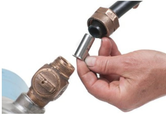
Figure 105 Stiffener slid inside PE tubing (BC Industry Training Authority, 2019). CC BY-NC-SA 4.0 ( https://creativecommons.org/licenses/by-nc-sa/4.0/ )
