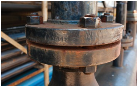
Figure 70 Example of assembled flanges (BC Industry Training Authority, 2019). CC BY-NC-SA 4.0 ( https://creativecommons.org/licenses/by-nc-sa/4.0/ )
