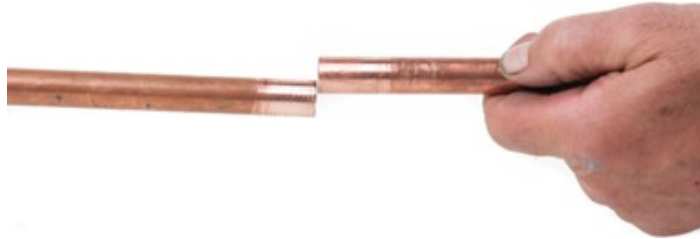
Figure 28 Pull one pipe end to one side (BC Industry Training Authority, 2019). CC BY-NC-SA 4.0 ( https://creativecommons.org/licenses/by-nc-sa/4.0/ )
