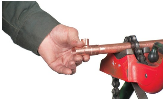
Figure 12 Insert and twist fitting fully (BC Industry Training Authority, 2019). CC BY-NC-SA 4.0 ( https://creativecommons.org/licenses/by-nc-sa/4.0/ )
