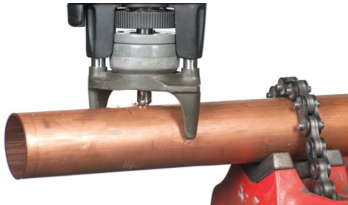
Figure 32 Position the drill tip and ensure a snug fit of the support legs (BC Industry Training Authority, 2019). CC BY-NC-SA 4.0 ( https://creativecommons.org/licenses/by-nc-sa/4.0/ )
