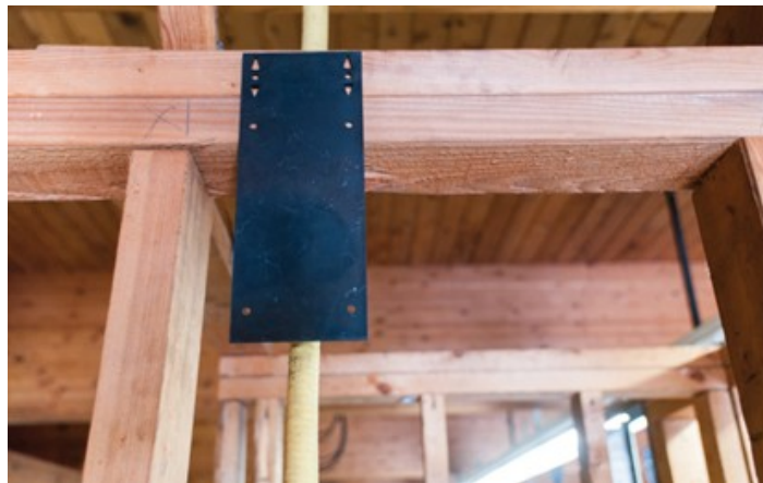
Figure 118 Striker plate applied at upper wall plates (BC Industry Training Authority, 2019). CC BY-NC-SA 4.0 ( https://creativecommons.org/licenses/by-nc-sa/4.0/ )
