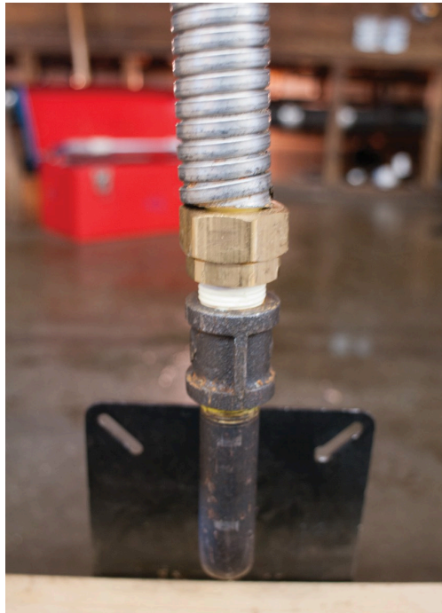
Figure 117 Floppy steel conduit installation (BC Industry Training Authority, 2019). CC BY-NC-SA 4.0 ( https://creativecommons.org/licenses/by-nc-sa/4.0/ )
