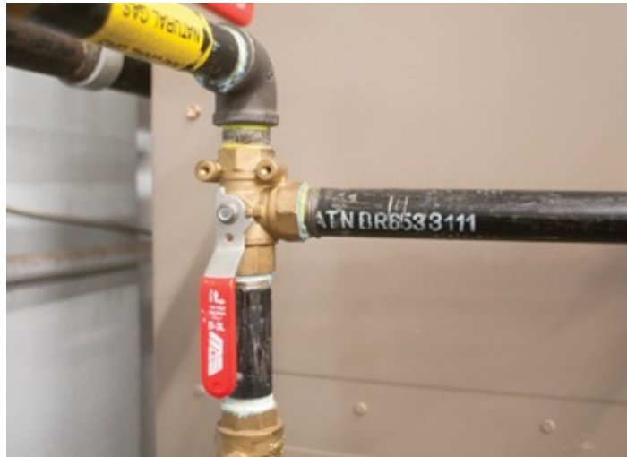
Figure 33 Three-port ball valve (BC Industry Training Authority, 2019). CC BY-NC-SA 4.0 ( https://creativecommons.org/licenses/by-nc-sa/4.0/ )
