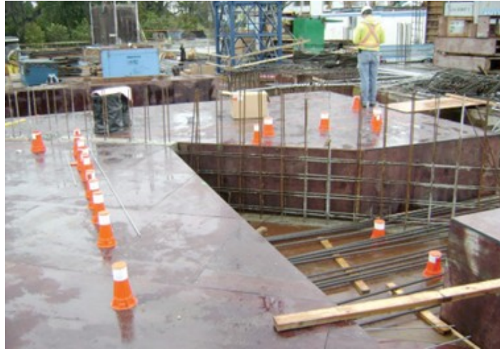
Figure 41 Pipe sleeves installed before reinforcing bar (BC Industry Training Authority, 2019). CC BY-NC-SA 4.0 ( https://creativecommons.org/licenses/by-nc-sa/4.0/ )
