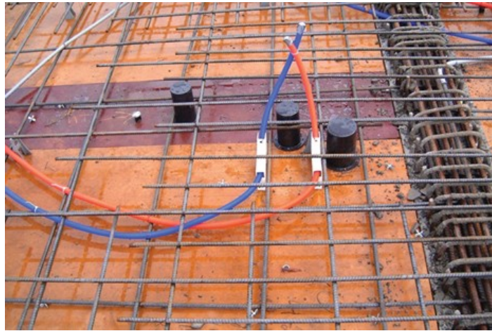
Figure 34 Formwork from above jack posts (BC Industry Training Authority, 2019). CC BY-NC-SA 4.0 ( https://creativecommons.org/licenses/by-nc-sa/4.0/ )
