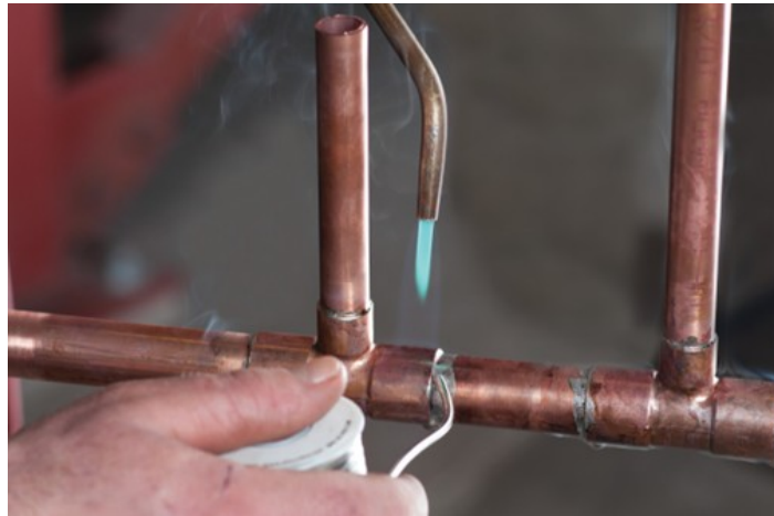
Figure 17 Applying solder (BC Industry Training Authority, 2019). CC BY-NC-SA 4.0 ( https://creativecommons.org/licenses/by-nc-sa/4.0/ )
