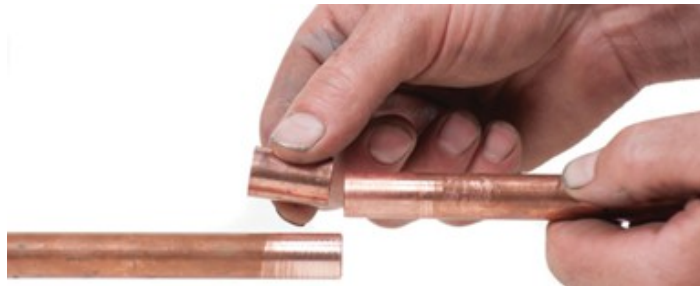
Figure 29 Slide the no-stop coupling over one end of the pipe (BC Industry Training Authority, 2019). CC BY-NC-SA 4.0 ( https://creativecommons.org/licenses/by-nc-sa/4.0/ )
