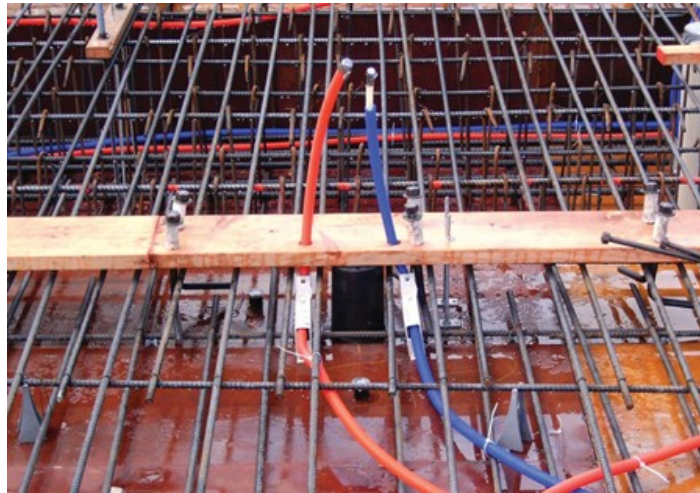
Figure 45 Positioning water pipes before pouring concrete (BC Industry Training Authority, 2019). CC BY-NC-SA 4.0 ( https://creativecommons.org/licenses/by-nc-sa/4.0/ )
