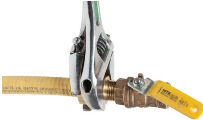
Figure 112 Tighten the fitting nut (BC Industry Training Authority, 2019). CC BY-NC-SA 4.0 ( https://creativecommons.org/licenses/by-nc-sa/4.0/ )
