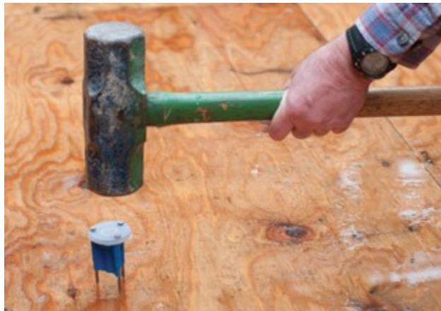
Figure 21 Installation (BC Industry Training Authority, 2019). CC BY-NC-SA 4.0 ( https://creativecommons.org/licenses/by-nc-sa/4.0/ )
