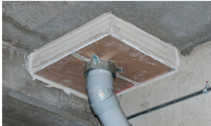
Figure 56 Gypsum board used in fire-blocking (BC Industry Training Authority, 2019). CC BY-NC-SA 4.0 ( https://creativecommons.org/licenses/by-nc-sa/4.0/ )
