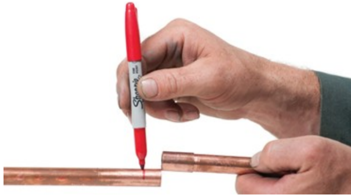
Figure 30 Mark the pipe (BC Industry Training Authority, 2019). CC BY-NC-SA 4.0 ( https://creativecommons.org/licenses/by-nc-sa/4.0/ )
