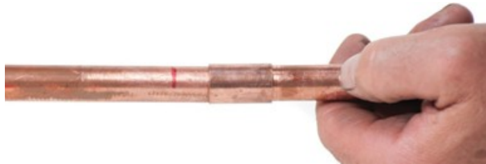
Figure 31 Realign the two pipes (BC Industry Training Authority, 2019). CC BY-NC-SA 4.0 ( https://creativecommons.org/licenses/by-nc-sa/4.0/ )
