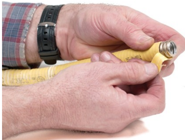
Figure 109 Strip the jacket (BC Industry Training Authority, 2019). CC BY-NC-SA 4.0 ( https://creativecommons.org/licenses/by-nc-sa/4.0/ )
