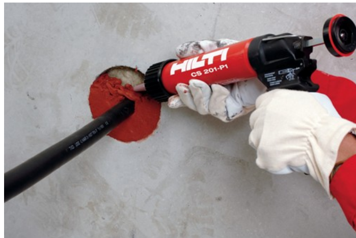
Figure 12 Latex firestop sealant installation (BC Industry Training Authority, 2019). CC BY-NC-SA 4.0 ( https://creativecommons.org/licenses/by-nc-sa/4.0/ )
