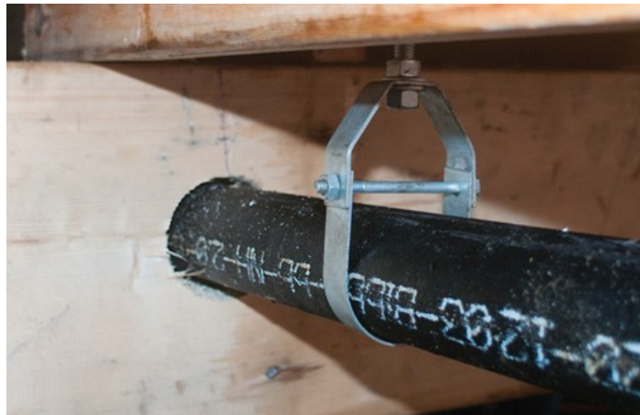
Figure 16 Proper drilling of holes and pipe support (BC Industry Training Authority, 2019). CC BY-NC-SA 4.0 ( https://creativecommons.org/licenses/by-nc-sa/4.0/ )
