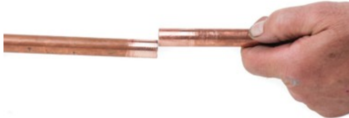
Figure 28 Pull one pipe end to one side (BC Industry Training Authority, 2019). CC BY-NC-SA 4.0 ( https://creativecommons.org/licenses/by-nc-sa/4.0/ )
