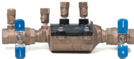
Figure 83 Double check valve assembly (BC Industry Training Authority, 2019). CC BY-NC-SA 4.0 ( https://creativecommons.org/licenses/by-nc-sa/4.0/ )
