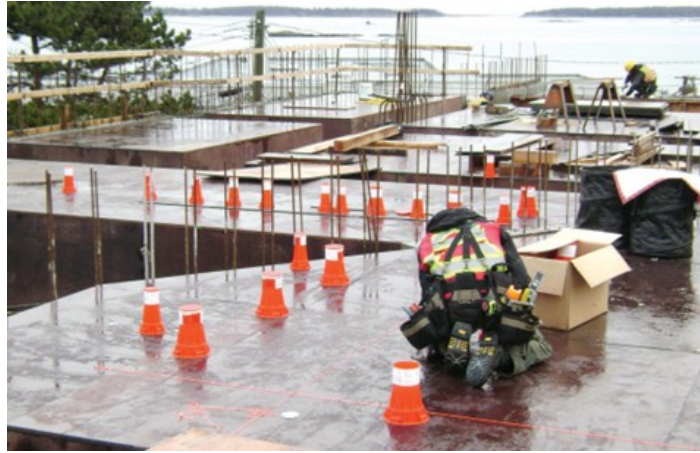
Figure 42 String lines to locate sleeve positions (BC Industry Training Authority, 2019). CC BY-NC-SA 4.0 ( https://creativecommons.org/licenses/by-nc-sa/4.0/ )
