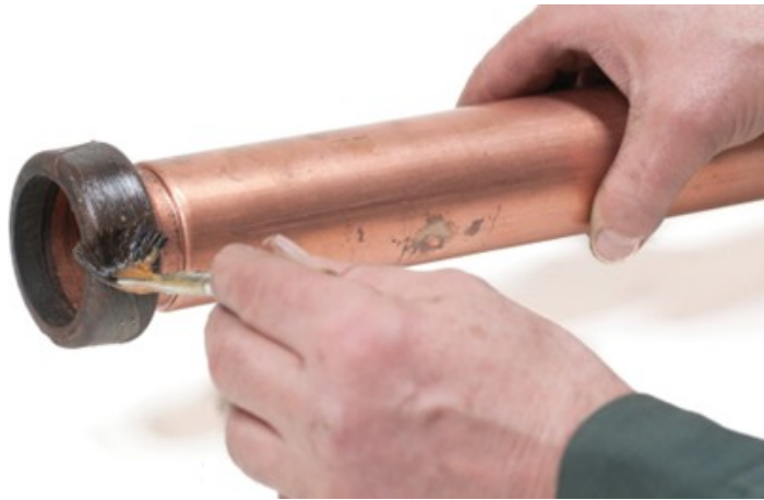
Figure 59 Apply lubrication (BC Industry Training Authority, 2019). CC BY-NC-SA 4.0 ( https://creativecommons.org/licenses/by-nc-sa/4.0/ )
