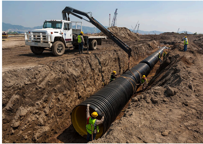
Figure 12 Hdpe pipe installation ( https://commons.wikimedia.org/wiki/File:Hdpe_pipe_installation.jpg ) (Tomascastelazo/Wikimedia Commons) CC BY-SA 3.0 ( https://creativecommons.org/licenses/by-sa/3.0/deed.en )
