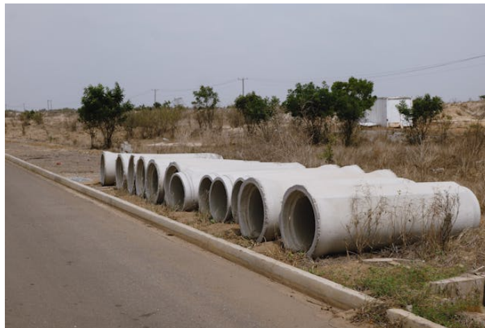
Figure 14 Industrial Concrete Pipes in Rural Landscape ( https://www.pexels.com/photo/industrial-concrete-pipes-in-rural-landscape-30762650/ ) (Andy Coffie/Pexels) Pexels License ( https://www.pexels.com/license/ )
