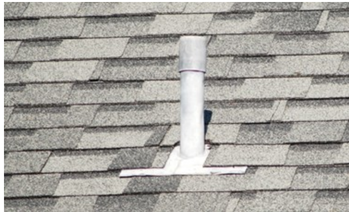
Figure 20 Roof plumbing vent penetration, lead flashing (BC Industry Training Authority, 2019). CC BY-NC-SA 4.0 ( https://creativecommons.org/licenses/by-nc-sa/4.0/ )
