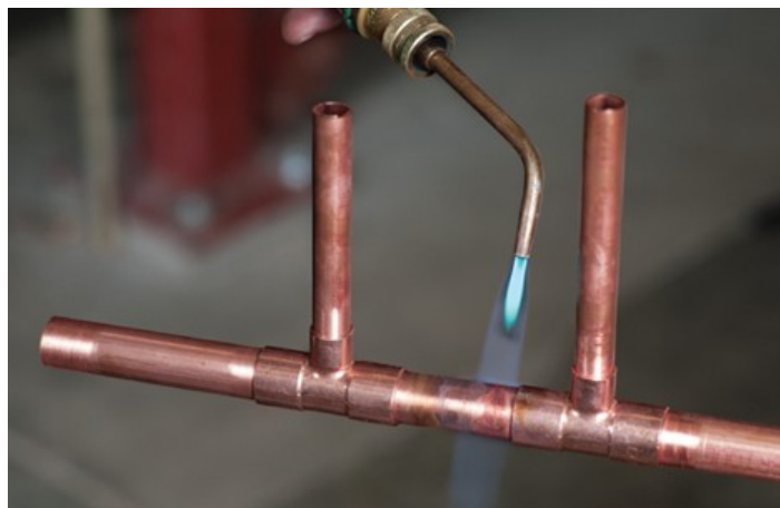
Figure 14 Preheat the tube (position 1 in Figure 15, right). (BC Industry Training Authority, 2019). CC BY-NC-SA 4.0 ( https://creativecommons.org/licenses/by-nc-sa/4.0/ )
