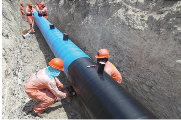
Figure 2 Moisture sealing a pipe casing (BC Industry Training Authority, 2019). CC BY-NC-SA 4.0 ( https://creativecommons.org/licenses/by-nc-sa/4.0/ )
