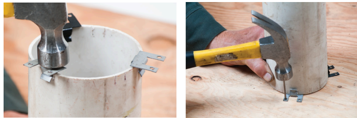
Figure 43 Attaching pipe sleeves using caddy clips (BC Industry Training Authority, 2019). CC BY-NC-SA 4.0 ( https://creativecommons.org/licenses/by-nc-sa/4.0/ )
