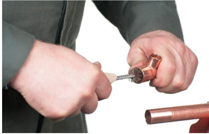
Figure 9 Clean inside fitting with fitting brush (BC Industry Training Authority, 2019). CC BY-NC-SA 4.0 ( https://creativecommons.org/licenses/by-nc-sa/4.0/ )
