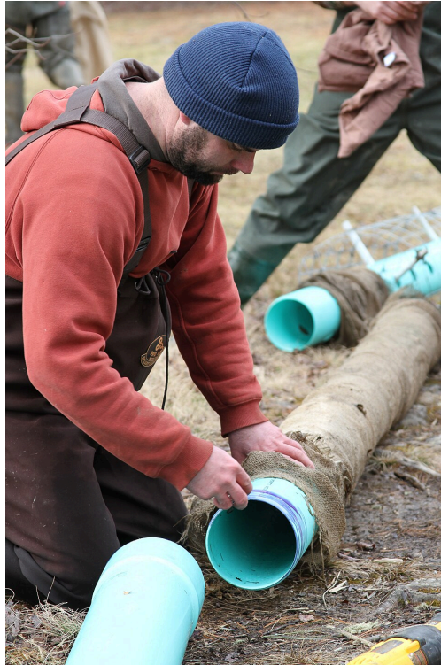
Figure 87 Glueing lengths of pipes ( https://commons.wikimedia.org/wiki/File:David_Caldwell_glueing_lengths_of_pipe_(12366938823).jpg ) (USFWS/Southeast/Wikimedia Commons) CC BY 2.0 ( https://creativecommons.org/licenses/by/2.0/deed.en )
