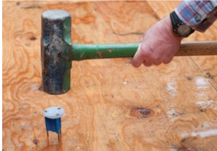
Figure 32 Pipe anchors (concrete hanger inserts) installed before the concrete is poured (BC Industry Training Authority, 2019). CC BY-NC-SA 4.0 ( https://creativecommons.org/licenses/by-nc-sa/4.0/ )
