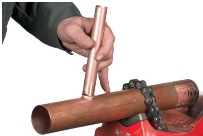
Figure 40 Align the dimples with the run of the tube (BC Industry Training Authority, 2019). CC BY-NC-SA 4.0 ( https://creativecommons.org/licenses/by-nc-sa/4.0/ )
