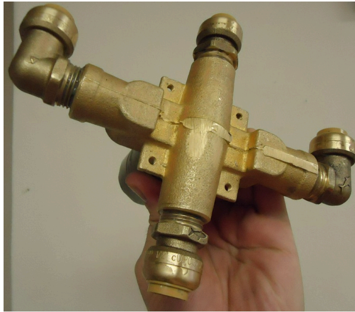
Figure 5 Diverter valve with PEX connections https://commons.wikimedia.org/wiki/File:Shower_project_new_diverter_valve_with_PEX_connections_added.jpg by (Tomwsulcer ( https://commons.wikimedia.org/w/index.php?title=User:Tomwsulcer&action=edit&redlink=1 )/Wikimedia Commons) CC0 1.0 ( https://creativecommons.org/publicdomain/zero/1.0/deed.en )
