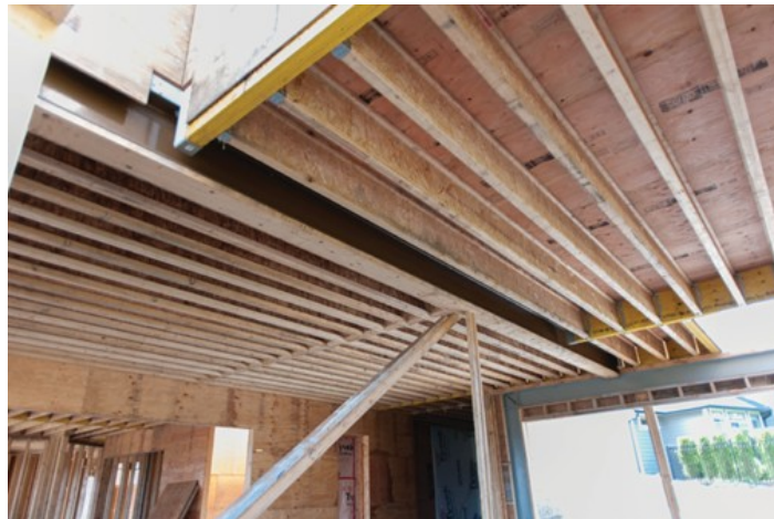
Figure 25 Steel I-beam supporting a wood deck (BC Industry Training Authority, 2019). CC BY-NC-SA 4.0 ( https://creativecommons.org/licenses/by-nc-sa/4.0/ )
