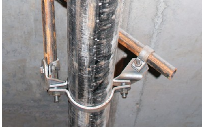
Figure 42 Sway brace attached to riser clamp and concrete structure (BC Industry Training Authority, 2019). CC BY-NC-SA 4.0 ( https://creativecommons.org/licenses/by-nc-sa/4.0/ )
