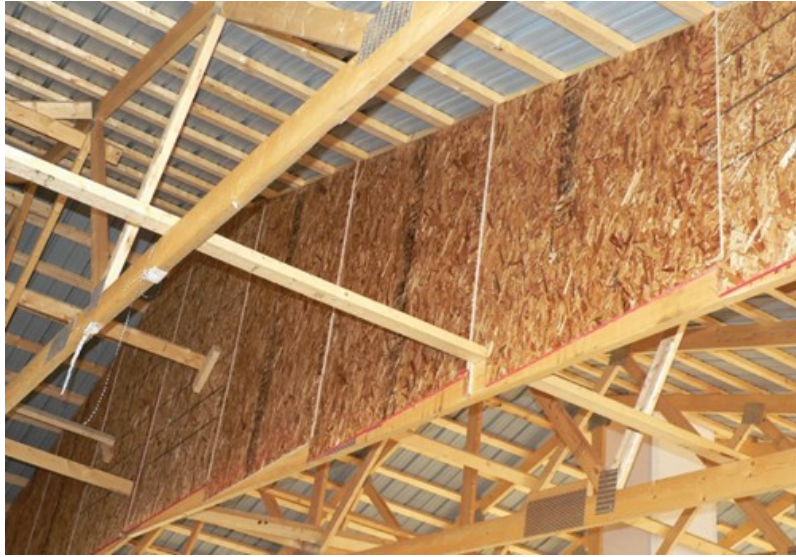
Figure 7 Attic fire block (BC Industry Training Authority, 2019). CC BY-NC-SA 4.0 ( https://creativecommons.org/licenses/by-nc-sa/4.0/ )
