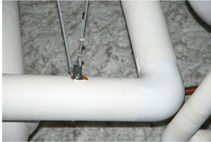
Figure 47 Cable attachment to pipe (BC Industry Training Authority, 2019). CC BY-NC-SA 4.0 ( https://creativecommons.org/licenses/by-nc-sa/4.0/ )
