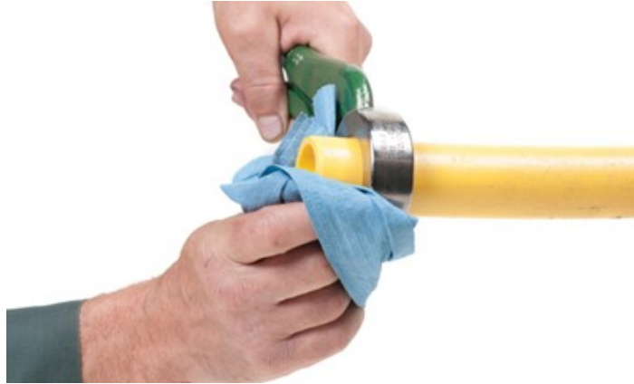
Figure 74 Cold-clamping ring being used in preparation for fusion welding hands-free without the fusion assembly (BC Industry Training Authority, 2019). CC BY-NC-SA 4.0 ( https://creativecommons.org/licenses/by-nc-sa/4.0/ )
