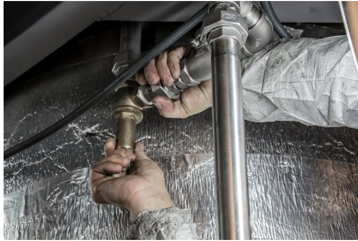
Figure 91 Plumber installs ( https://www.pexels.com/photo/plumber-installs-pipe-fittings-6419128/ ) (Anıl Karakaya/Pexels) Pexels license ( https://www.pexels.com/license/ )
