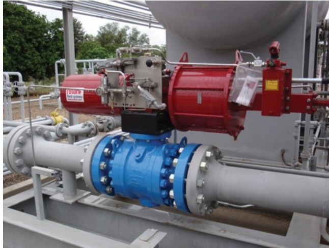
Figure 11 Hydraulically operated ball valve (BC Industry Training Authority, 2019). CC BY-NC-SA 4.0 ( https://creativecommons.org/licenses/by-nc-sa/4.0/ )
