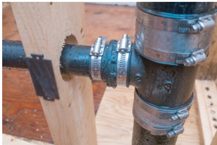
Figure 19 Protection plate on a stud over an ABS pipe (BC Industry Training Authority, 2019). CC BY-NC-SA 4.0 ( https://creativecommons.org/licenses/by-nc-sa/4.0/ )
