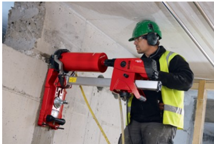
Figure 47 Diamond drill coring (BC Industry Training Authority, 2019). CC BY-NC-SA 4.0 ( https://creativecommons.org/licenses/by-nc-sa/4.0/ )
