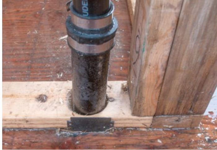
Figure 18 Correct use of pipe protection plates (BC Industry Training Authority, 2019). CC BY-NC-SA 4.0 ( https://creativecommons.org/licenses/by-nc-sa/4.0/ )
