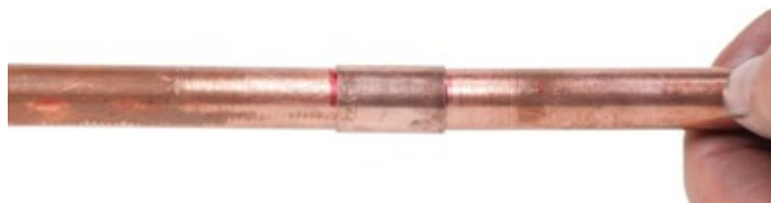
Figure 32 Slide the no-stop coupling back to the mark on the pipe (BC Industry Training Authority, 2019). CC BY-NC-SA 4.0 ( https://creativecommons.org/licenses/by-nc-sa/4.0/ )
