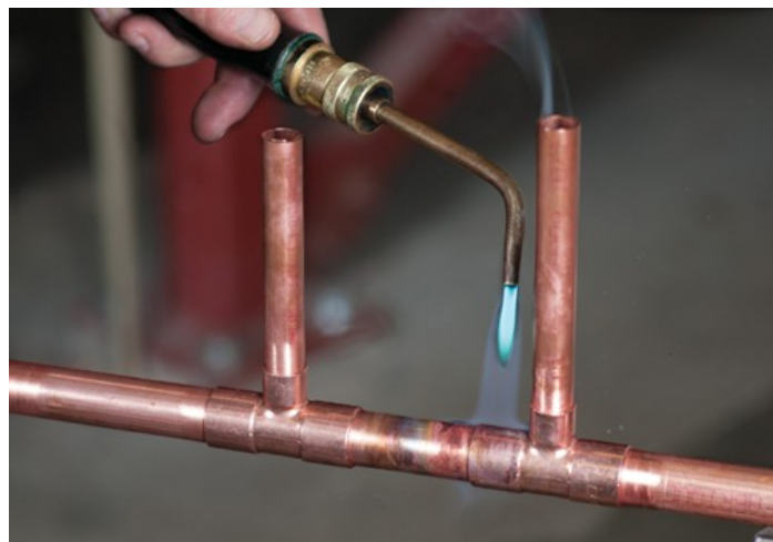
Figure 16 Preheat the fitting cup (position 2) (BC Industry Training Authority, 2019). CC BY-NC-SA 4.0 ( https://creativecommons.org/licenses/by-nc-sa/4.0/ )
