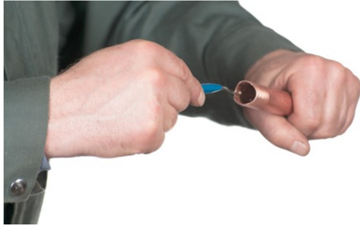
Figure 37 Ream the branch tube end (BC Industry Training Authority, 2019). CC BY-NC-SA 4.0 ( https://creativecommons.org/licenses/by-nc-sa/4.0/ )
