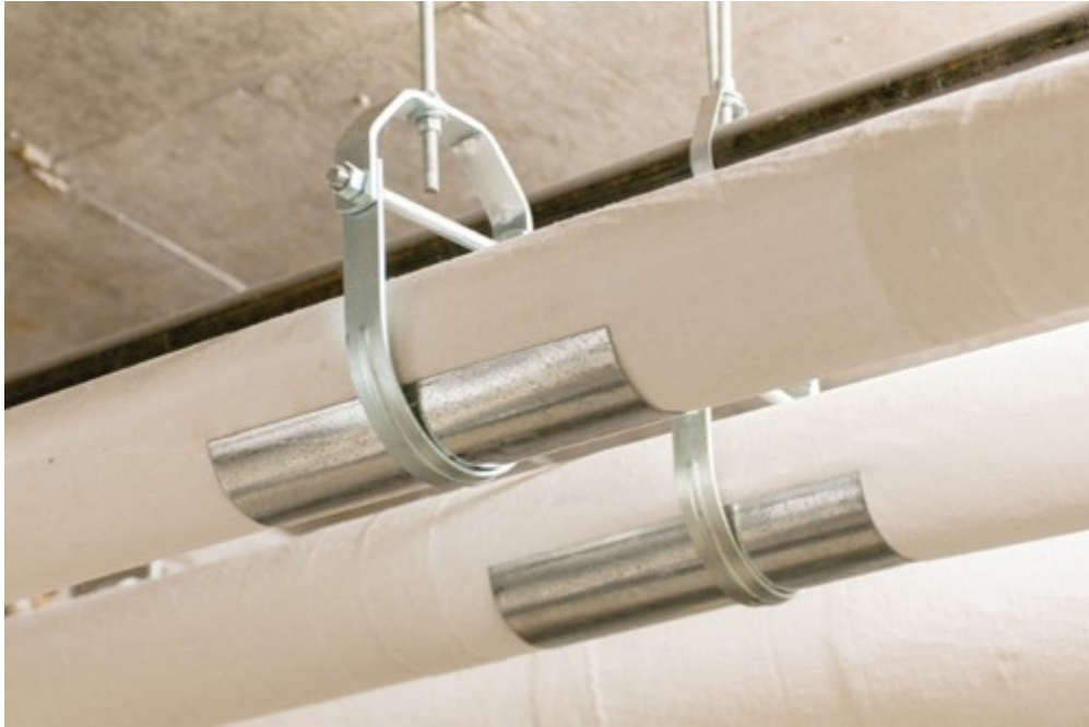
Figure 13 Sliding pipe saddle installation (BC Industry Training Authority, 2019). CC BY-NC-SA 4.0 ( https://creativecommons.org/licenses/by-nc-sa/4.0/ )
