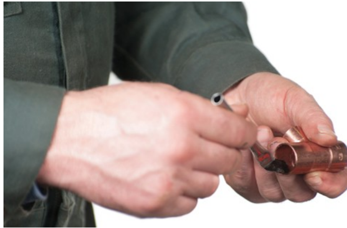
Figure 11 Flux the fitting (do not overload the fitting with flux) (BC Industry Training Authority, 2019). CC BY-NC-SA 4.0 ( https://creativecommons.org/licenses/by-nc-sa/4.0/ )
