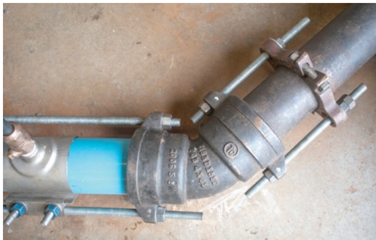
Figure 124 Ductile iron push-on joint pipe fitting (BC Industry Training Authority, 2019). CC BY-NC-SA 4.0 ( https://creativecommons.org/licenses/by-nc-sa/4.0/ )
