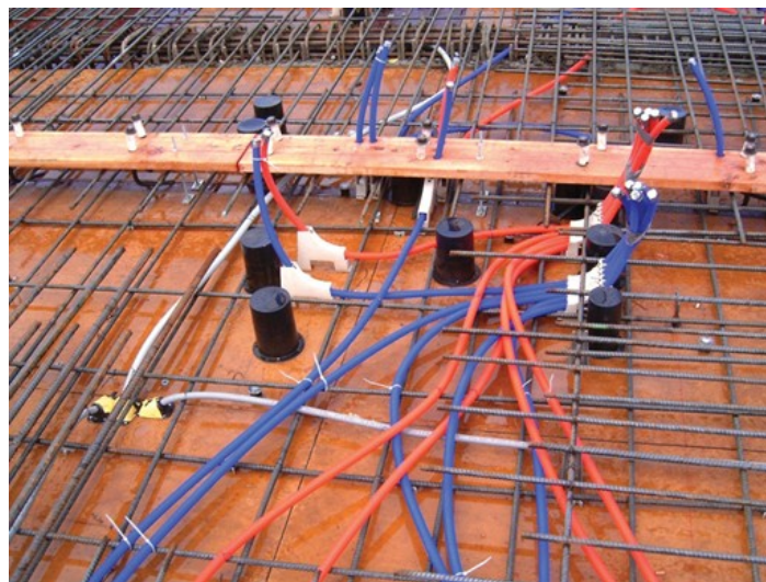
Figure 30 Rebar, electrical conduit, pipes, and pipe sleeves ready to be buried in concrete (BC Industry Training Authority, 2019). CC BY-NC-SA 4.0 ( https://creativecommons.org/licenses/by-nc-sa/4.0/ )
