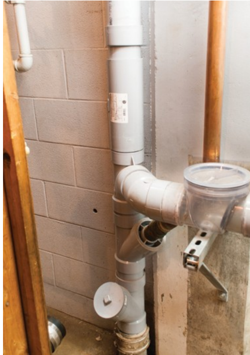
Figure 41 Installed PVC expansion joint (BC Industry Training Authority, 2019). CC BY-NC-SA 4.0 ( https://creativecommons.org/licenses/by-nc-sa/4.0/ )
