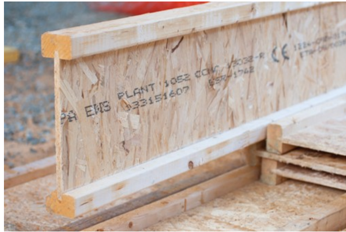
Figure 8 Wood I-beam type joist components (BC Industry Training Authority, 2019). CC BY-NC-SA 4.0 ( https://creativecommons.org/licenses/by-nc-sa/4.0/ )
