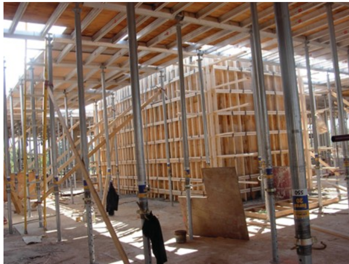
Figure 33 First floor formwork (BC Industry Training Authority, 2019). CC BY-NC-SA 4.0 ( https://creativecommons.org/licenses/by-nc-sa/4.0/ )
