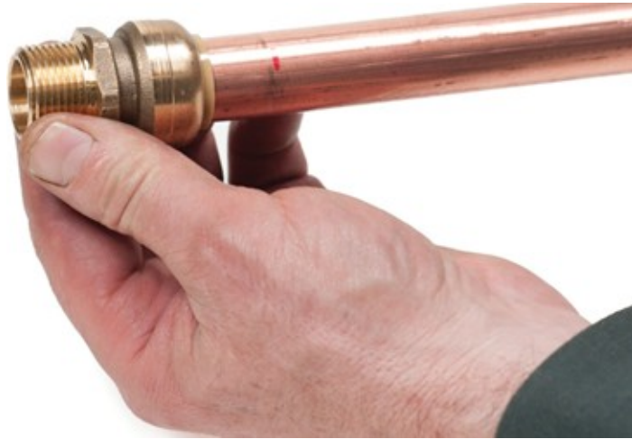
Figure 48 Align tube and fitting, push and twist together (BC Industry Training Authority, 2019). CC BY-NC-SA 4.0 ( https://creativecommons.org/licenses/by-nc-sa/4.0/ )
