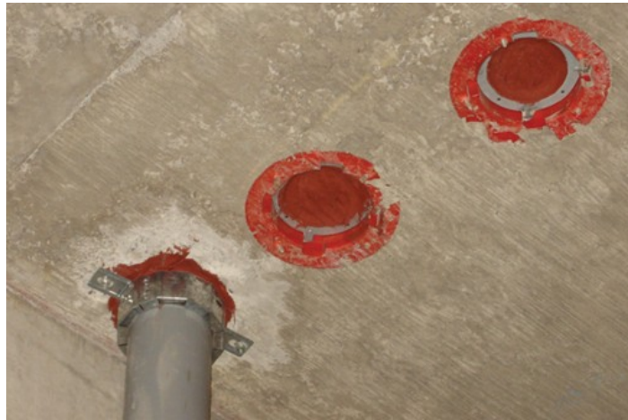
Figure 53 Fire-stop application (BC Industry Training Authority, 2019). CC BY-NC-SA 4.0 ( https://creativecommons.org/licenses/by-nc-sa/4.0/ )
