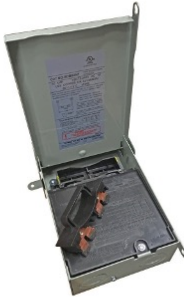
Figure 15 Disconnect switch (BC Industry Training Authority, 2019). CC BY-NC-SA 4.0
