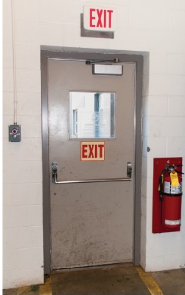
Figure 7 Fire extinguisher near exit (BC Industry Training Authority, 2019). CC BY-NC-SA 4.0 ( https://creativecommons.org/licenses/by-nc-sa/4.0/ )
