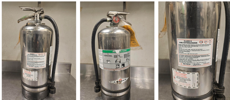
Figure 3 Class K fire extinguisher (Daniel Abdulai/TRU Open Press). CC BY-NC-SA ( https://creativecommons.org/licenses/by-nc-sa/4.0/deed.en )
