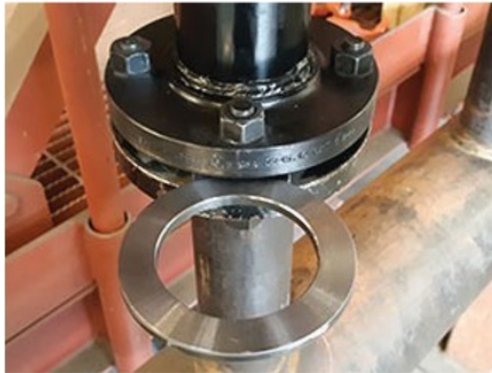
Figure 11 Spectacle blind installed (BC Industry Training Authority, 2019). CC BY-NC-SA 4.0 ( https://creativecommons.org/licenses/by-nc-sa/4.0/ )
