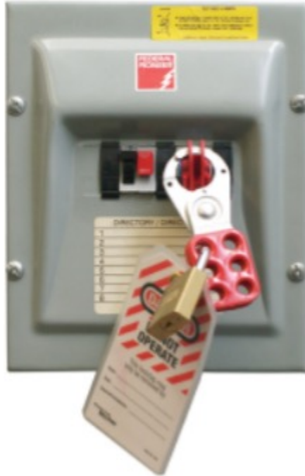
Figure 1 Safety switch locked out (BC Industry Training Authority, 2019). CC BY-NC-SA 4.0 ( https://creativecommons.org/licenses/by-nc-sa/4.0/ )
