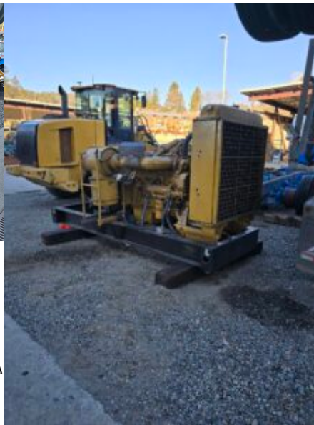
Figure 4b. Engine and generator unit secured on cribbing blocks to maintain elevation and prevent shifting during servicing. (Audrey Curran/TRU Open Press) CC BY-NC-SA 4.0 ( https://creativecommons.org/licenses/by-nc-sa/4.0/ )
