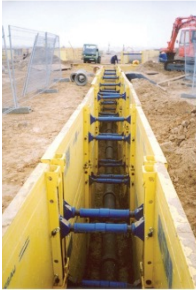
Figure 1 Prefabricated hydraulic shoring (Sbhirus/Wikimedia Commons) CC BY SA 3.0 ( https://creativecommons.org/licenses/by-sa/3.0/deed.en )
