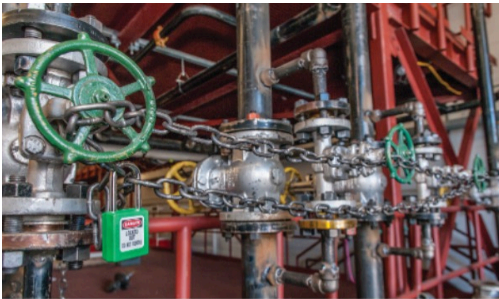
Figure 3 Chains used to lock out valve handles (BC Industry Training Authority, 2019). CC BY-NC-SA 4.0 ( https://creativecommons.org/licenses/by-nc-sa/4.0/ )
