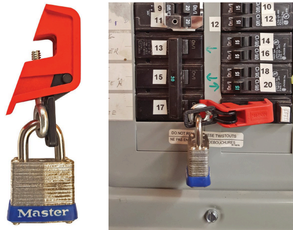
Figure 6 Breaker lockouts (BC Industry Training Authority, 2019). CC BY-NC-SA 4.0 ( https://creativecommons.org/licenses/by-nc-sa/4.0/ )
